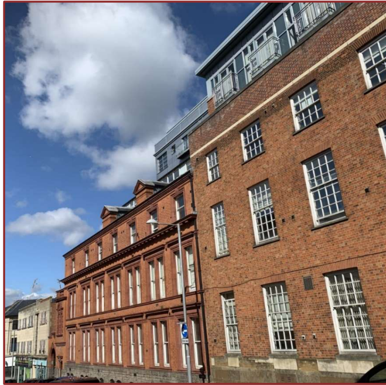
West facing elevations to Castle Exchange consisting of glazing, masonry and curtain walling system
