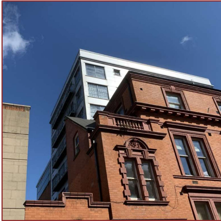
North West facing elevations to Castle Exchange consisting of balconies and aluminium curtain walling system
